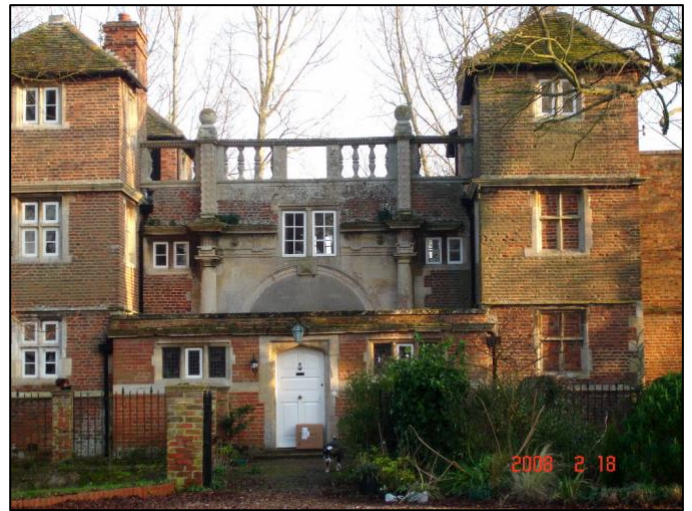
Photo 1. The gatehouse, of narrow red brick with stone dressings, showing 1904 alteration to entrance. Ann Colbert.
