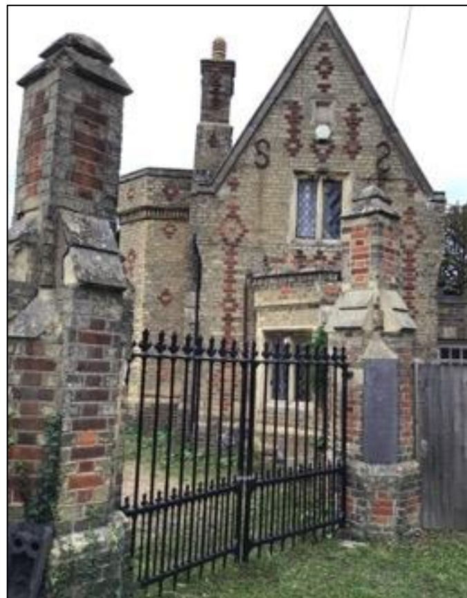
Figure 9. Gothic lodge, showing a 'two-storey Elizabethan Tudor-style lodge (listed grade II) built of grey gault brick with red diapering and stone dressings under a roof of octagonal slates' (Historic England Listing 1126200). Loudon (1843, p116, Fig. 56) shows the roof slate detail.
