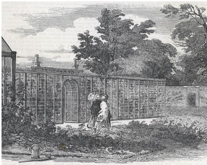
Figure 14. Ewing's glass wall, designed for the garden of the Royal Horticultural Society at Chiswick. Image from The Illustrated London News , 28 August 1852.
