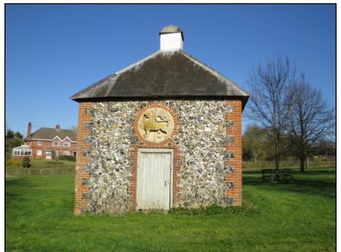
The 18C flint dovecote with red brick dressings, one of the remaining estate buildings. The carved heraldic lion is much earlier and may have come from the old hall.
