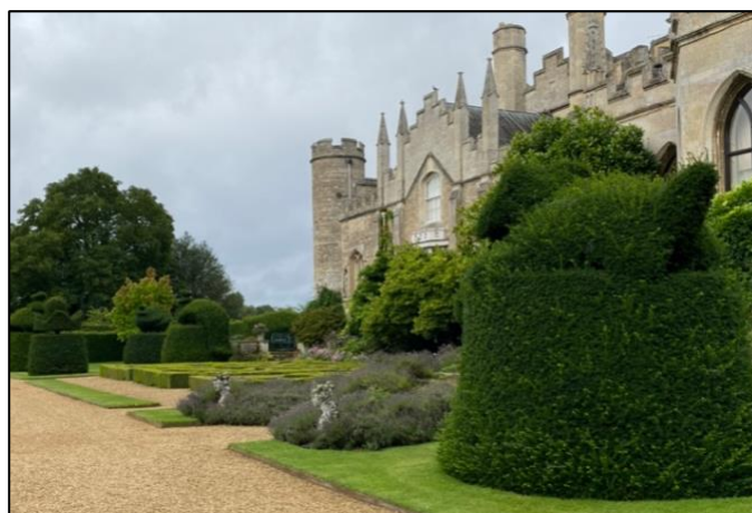
Figure 1. The SE elevation of Elton Hall showing some of the range of architectural styles looking out over parterres and clipped greens. Photo by Sarah Hundleby.
